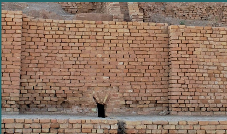
Drainage System in the Tchogha Zanbil ziggurat (2nd millennium BC). Photo by Masoud Nakhaei, 2015.
